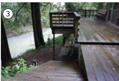
Figure 45: Deck and stairs looking east
