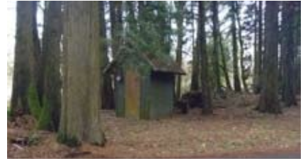
Figure 23: existing well house on "White" property.
