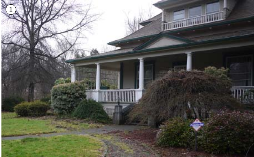
figure 35: Front (north side) of the Schacht House
