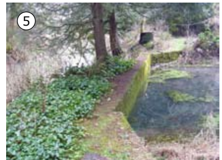
Figure 49: Concrete weir and pond
