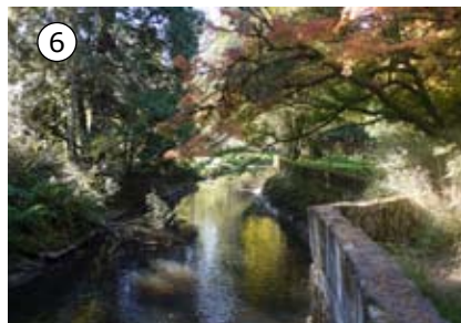
Figure 30 - 31: Stream bank armoring
