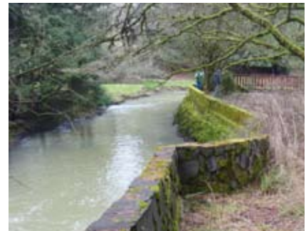
Figure 3: Johnson Creek bank armoring.
