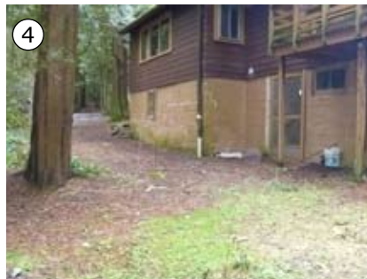
Figure 46: East side of Allesina house, looking south
