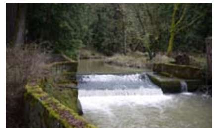
Figure 10: Water control structure
